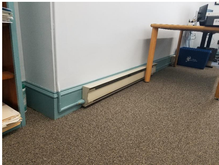
Electric Baseboard Heating Element
