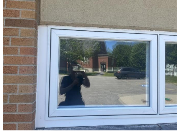
Figure 9: Typical aluminum projected window at the gymnasium.
