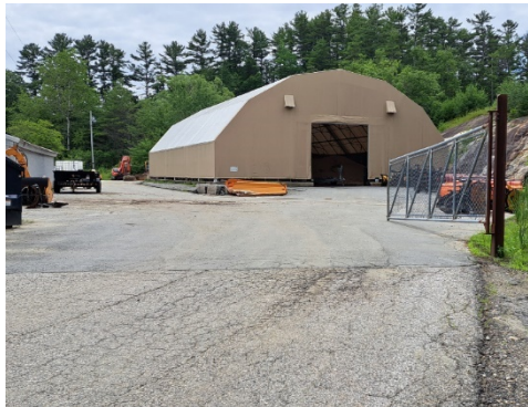
Gate at northeast corner
