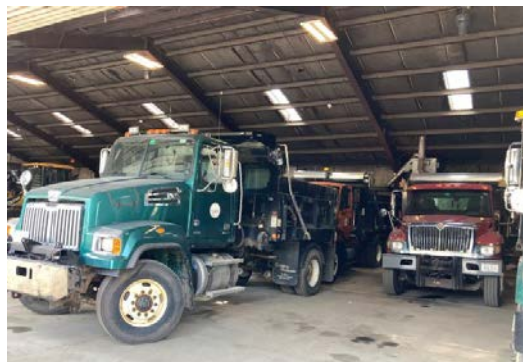
Faced Insulation Ceiling in Garage
