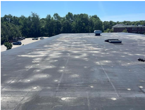
Figure 12: Overall view of the roof.
