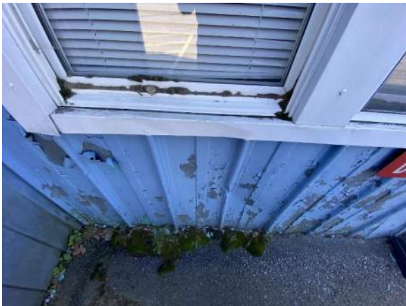
Figure 10: Algae and vegetative growth at windowsill.
