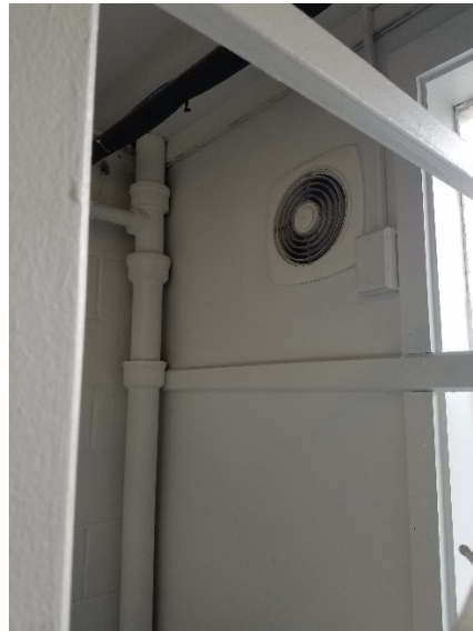
Wall Mounted Exhaust Fan
