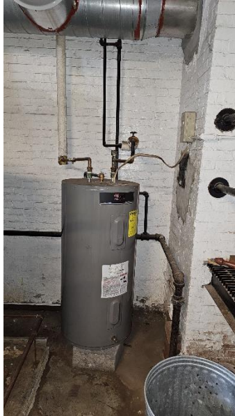
Electric Water Heater
