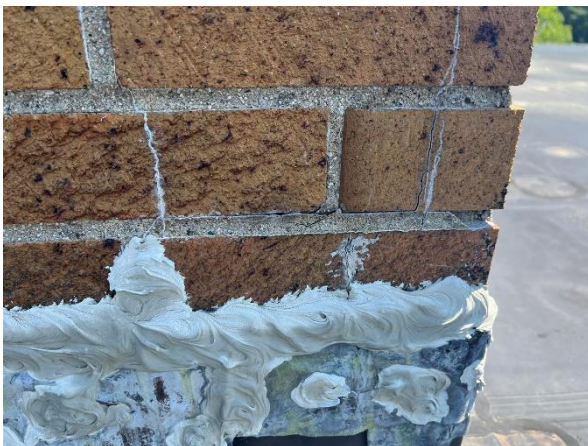
Figure 14: Sealant repairs at the chimney flashing.
