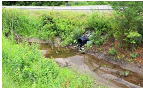
Drainage swale at road
