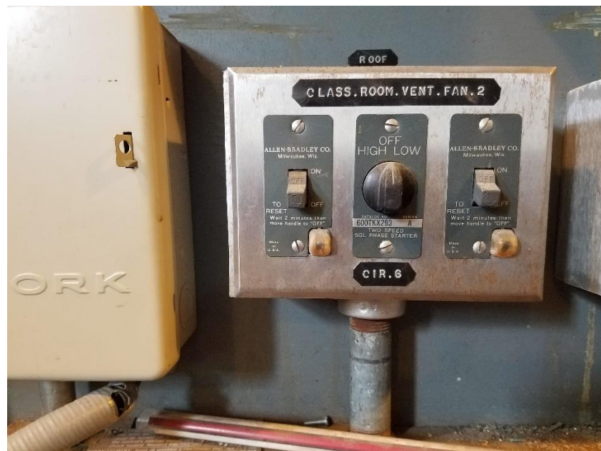
Motor Rated Manual Switches
