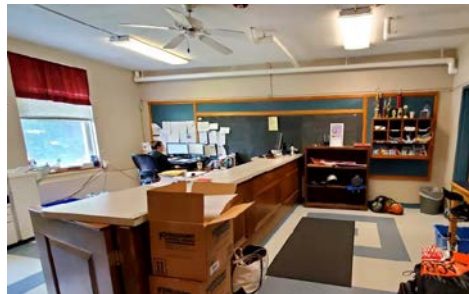
Classroom GPDW Ceiling
