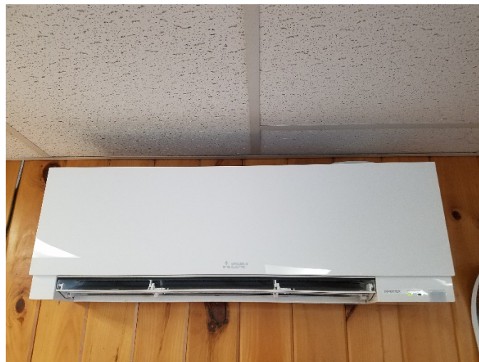
Wall Mounted Indoor Evaporator
