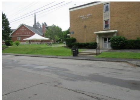
Slope at front of building, Sheridan Road
