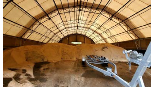
Salt Barn Interior
