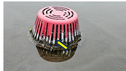
Roof Drain Set Above Roof
