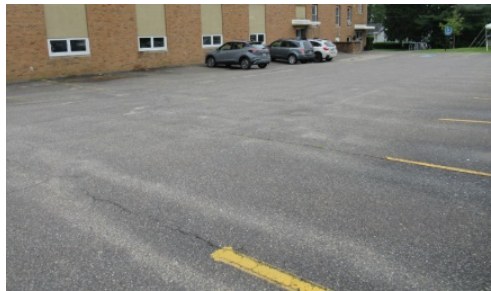
Pavement at east parking lot
