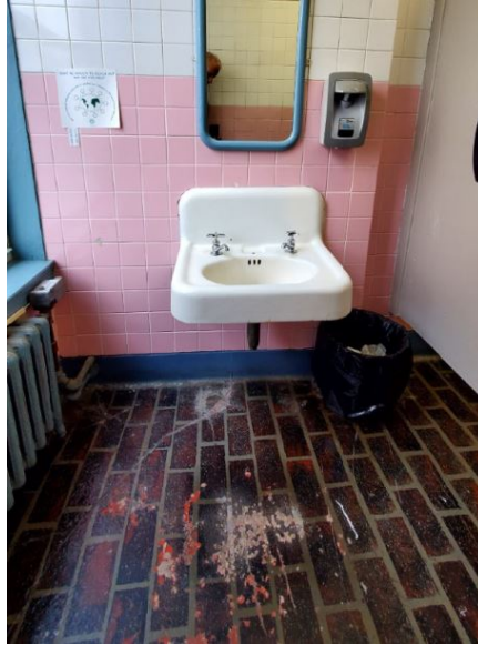
Toilet Room Flooring
