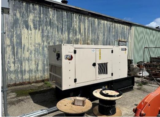
New generator being installed
