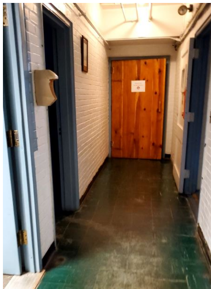
Basement Corridor Walls
