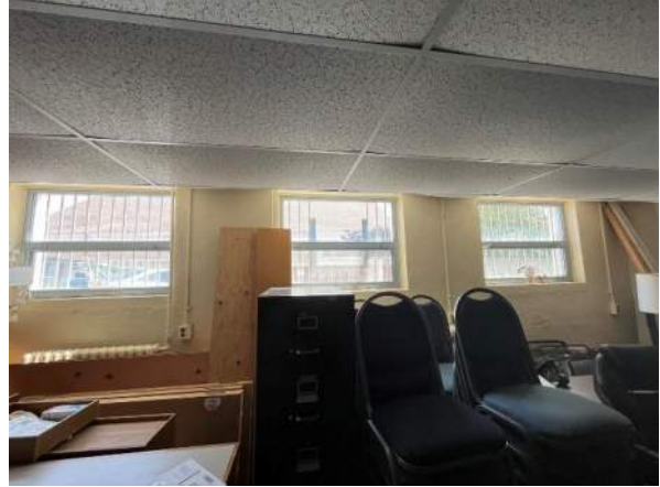
Figure 17: Projected windows at the basement level.
