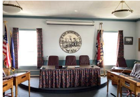
12" Acoustical Ceiling Tiles
