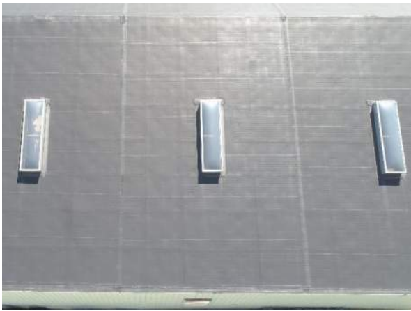
Figure 12: EPDM roofing system with dome skylights.
