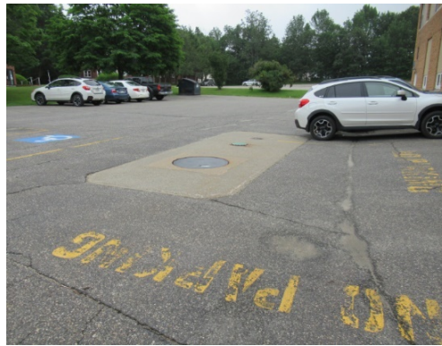
Overall site slope looking southeasterly
