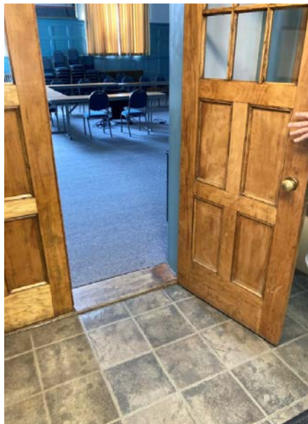
Door, Hardware at Meeting Room
