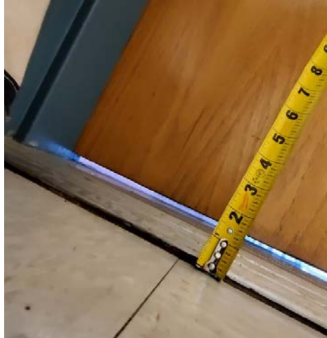
Toilet Room Threshold
