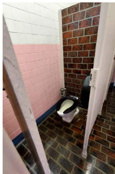
Toilet Room Ceramic Tile Walls, Base
