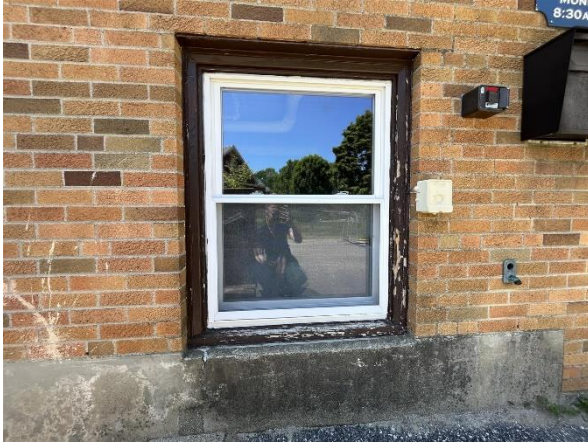
Figure 8: Typical aluminum hung window at original wood window frame.
