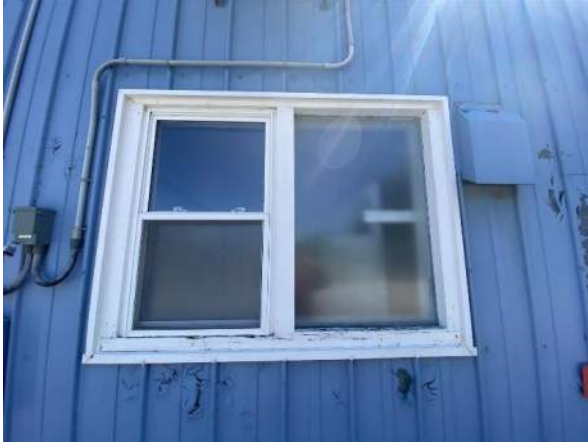
Figure 8: Typical existing window at wood frame.
