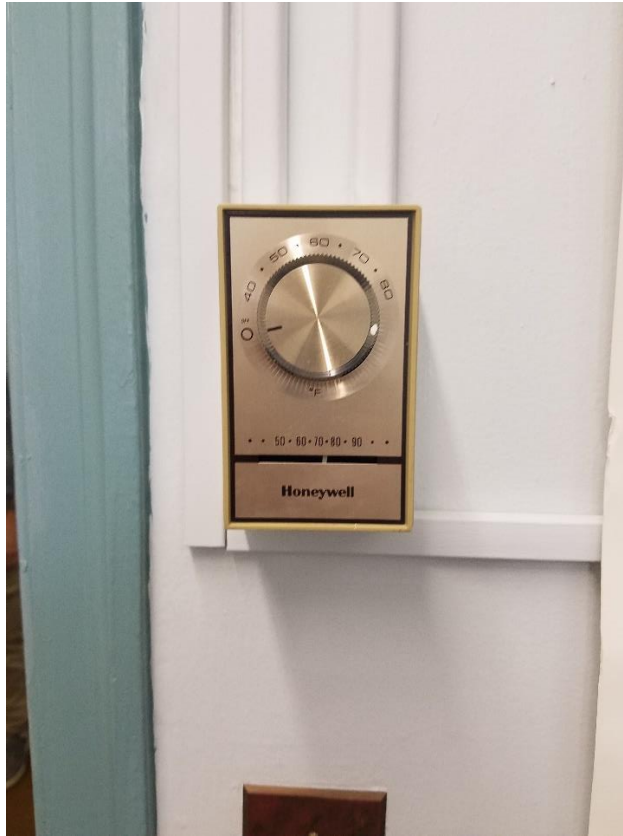
Electric Stand-Alone Thermostat
