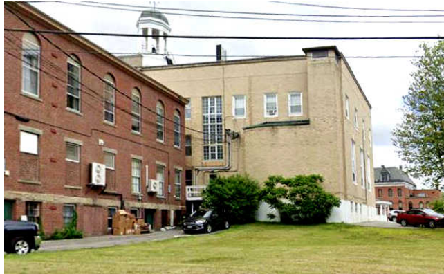
Overhead Power Lines
