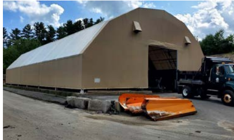
Salt Barn Exterior
