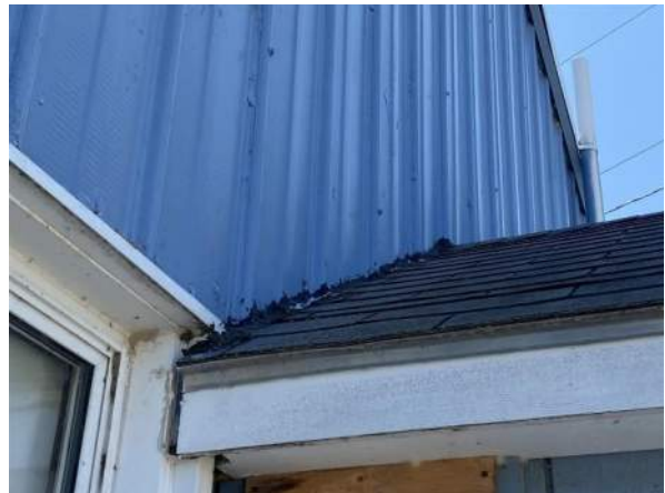
Figure 15: Asphalt shingle roof with asphalt roof cement at the metal panel wall transition.
