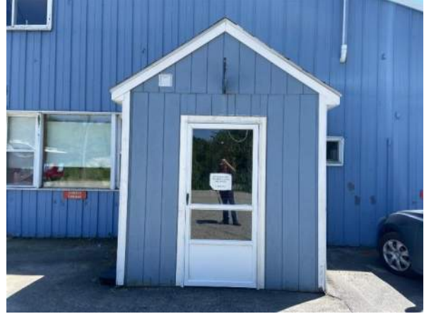
Figure 7: Wood siding at entry vestibule.
