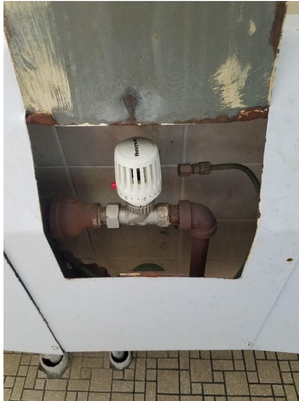
Self-Contained Steam Radiator Valve
