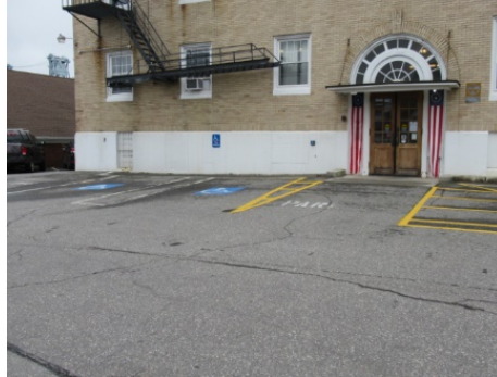
HC Parking and signage at main entrance
