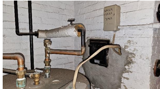
Two Water Service Pipes
