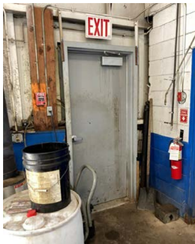
Door in Shop Area
