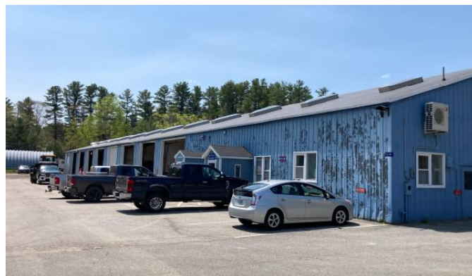
Building Exterior Condition
