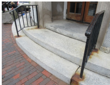
Front Street Entrance
