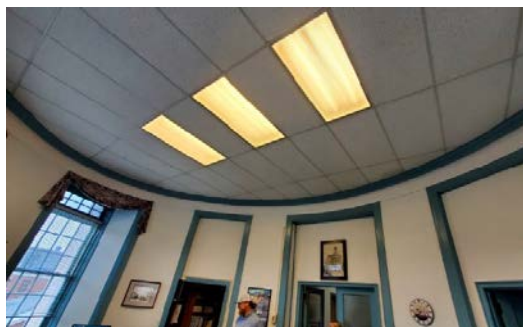
2x4 Ceiling Tiles in Office
