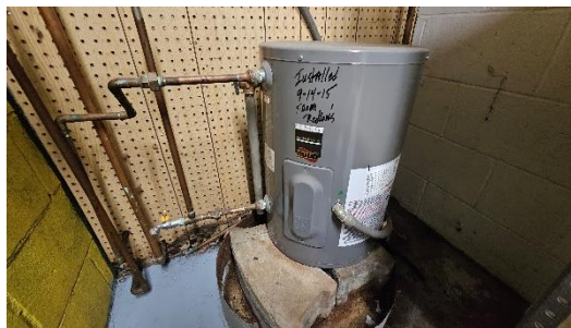
Electric Water Heater
