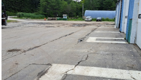
Bituminous pavement at service bays
