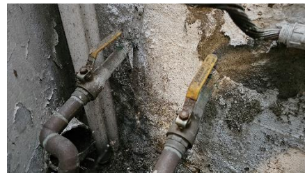
Two Water Service Pipes
