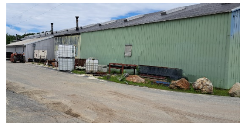
Storage area at rear of building
