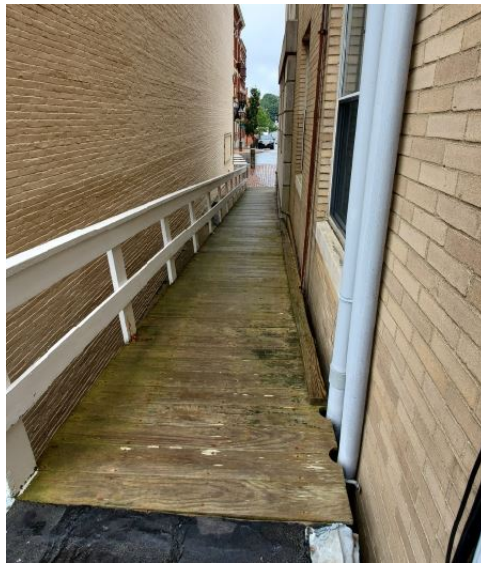
South Side Ramp
