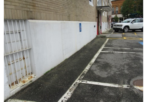
HC Parking at wall
