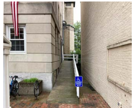
Alleyway with Limited Visibility
