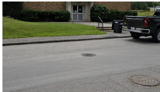
Combined Storm/Sewer Access Cover in Sheridan Road
