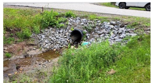
West driveway culvert
