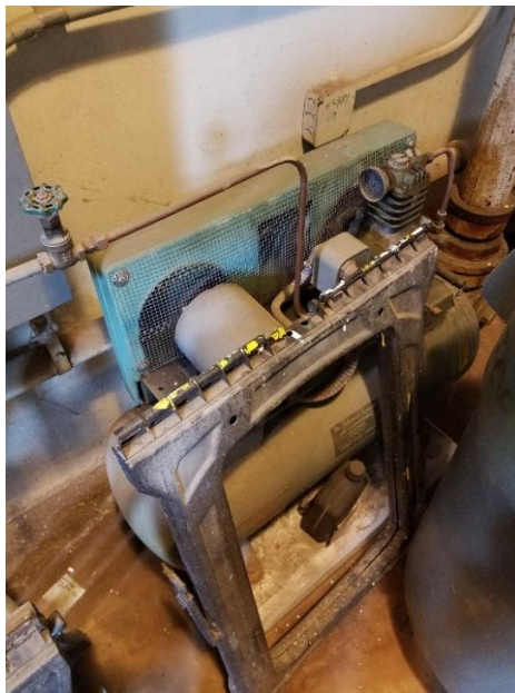
Pneumatic Air Compressor
