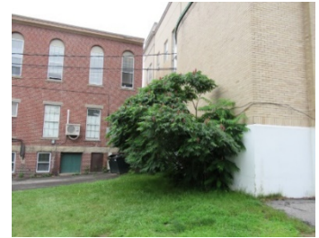
Slope behind building
