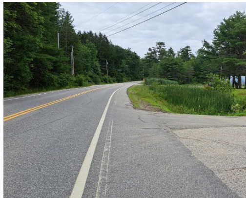
Sight distance to west
