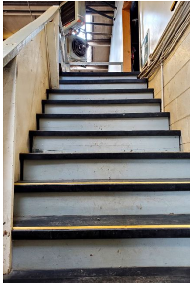
Stair to Mezzanine
