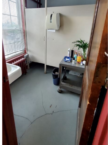
Toilet Room Flooring
