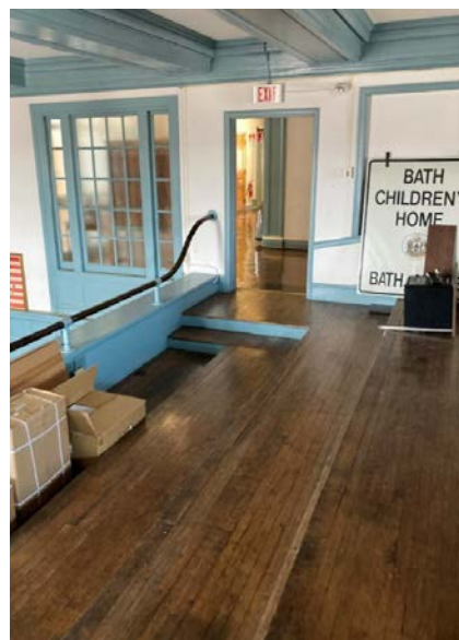
Balcony Wooden Flooring
