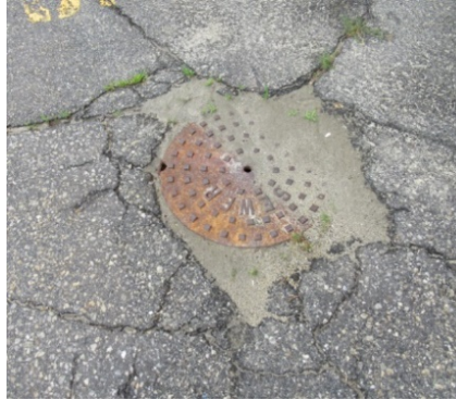
Sewer manhole cover
