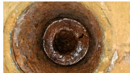
Interior of Pipe in Floor Cleanout
