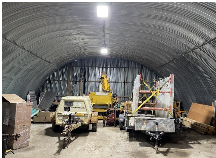
Storage shed interior.
