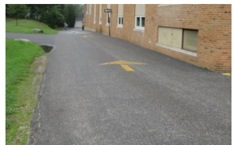
Pavement at west driveway
