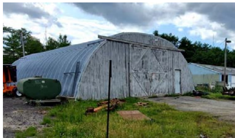
Storage Building Exterior
