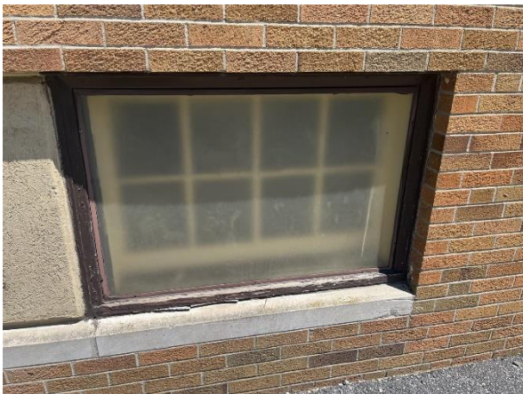
Figure 10: Original wood window with exterior mounted storm window.
