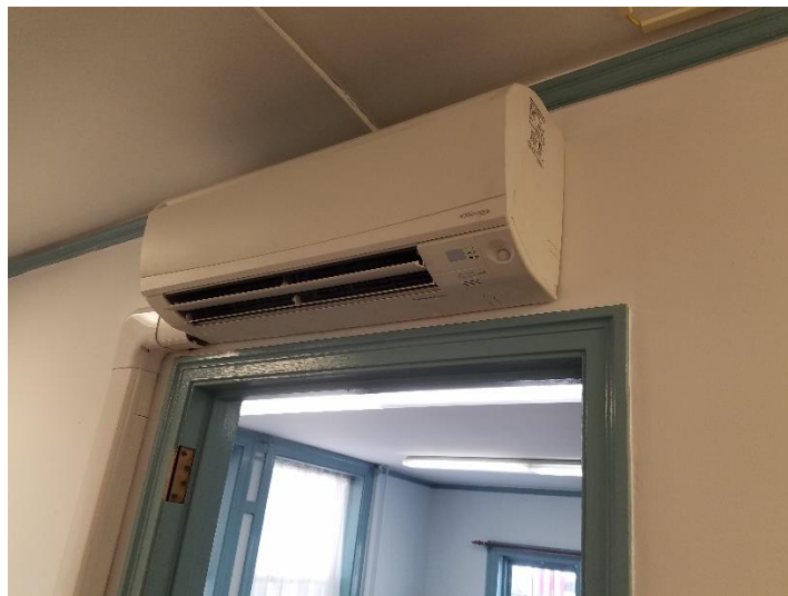
Wall Mounted Evaporator Unit
