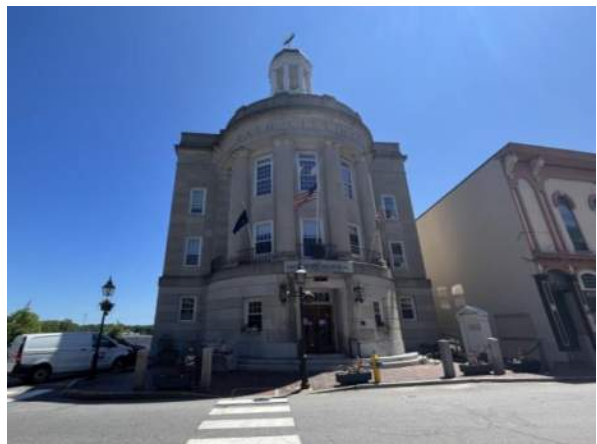
Figure 1: Bath City Hall west elevation.
