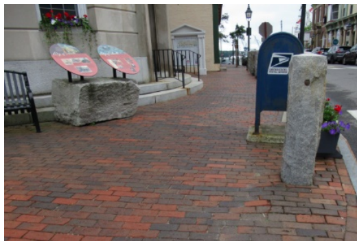
Brick pavement at Front Street
