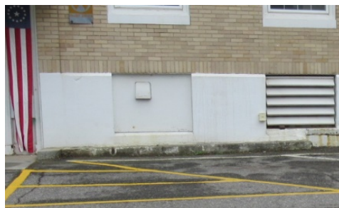
Curb at head of parking
